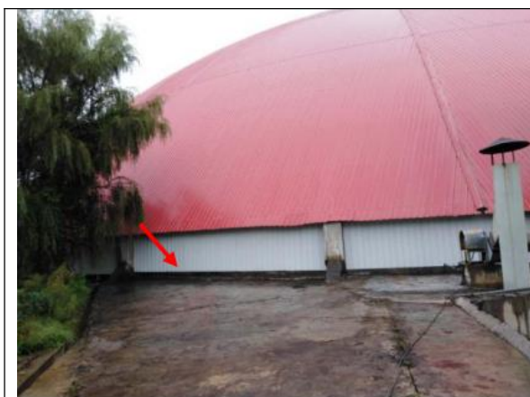
对煤预均化库底部实施了全封闭
